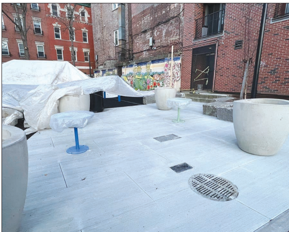
Plaza and table installation in progress.
