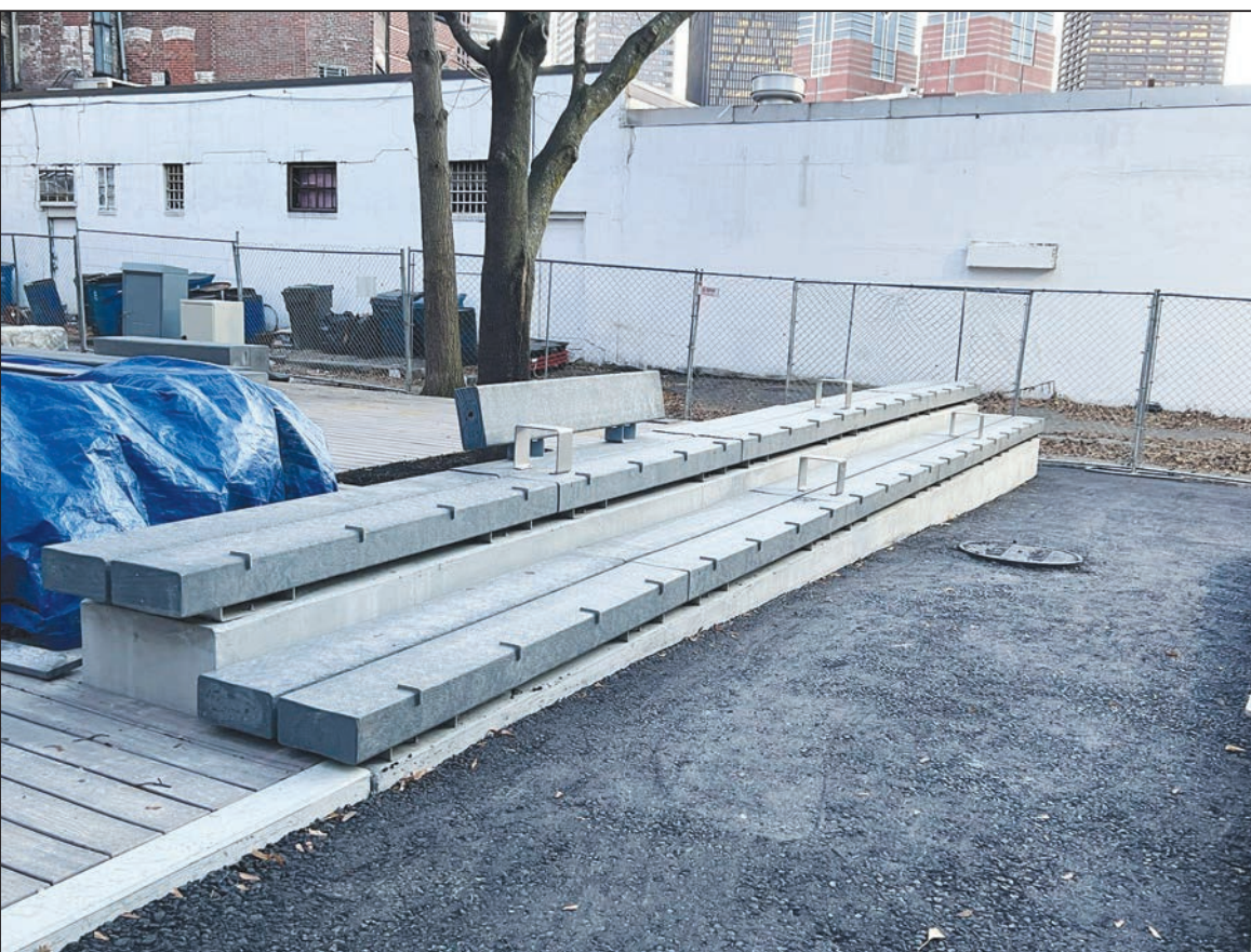
Custom benches are being constructed.
