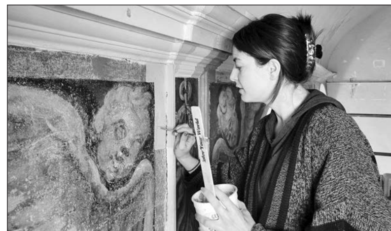
A worker painstakingly removes layers of white paint to partially uncover one of the angels painted in 1727.
