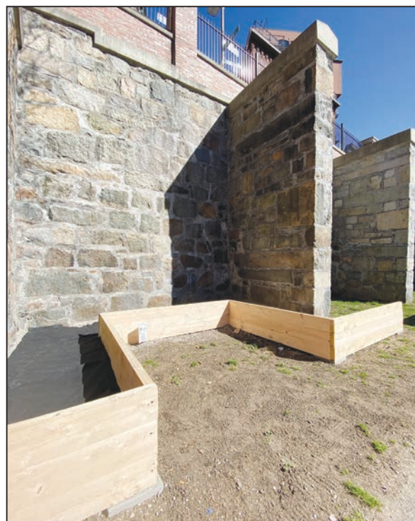
Community garden construction at DeFilippo Park is currently underway.
